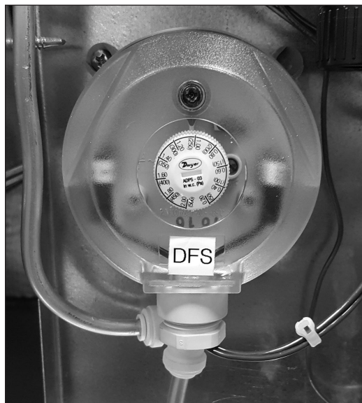
Figure 26.3 - Dirty Filter Pressure Switch
