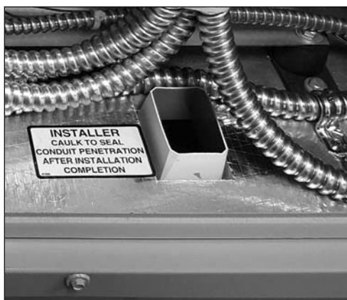
Figure 11.2 - Floor Wiring Chase
